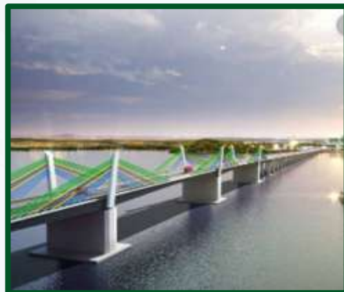
Financed construction of Busisi bridge across lake Victoria – USD 256 Mln
