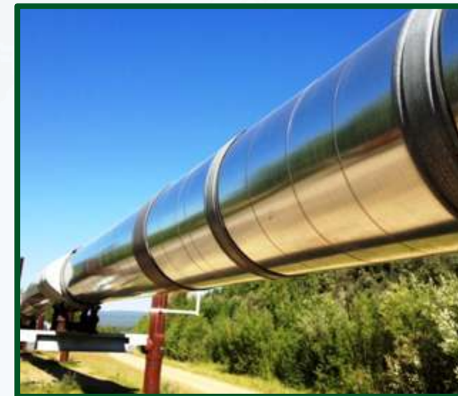
Financed Hoima Tanga crude oil project – USD 152
